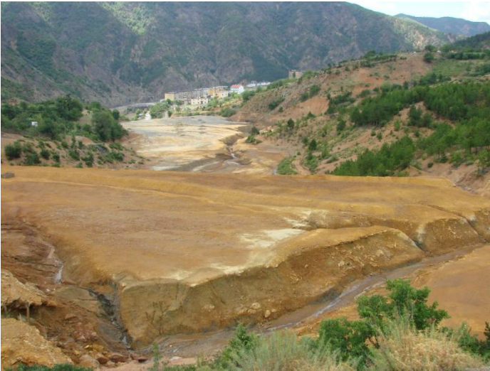
PHOTO OF THE DAM, FUSHE ARREZ TREATMENT PLAN
